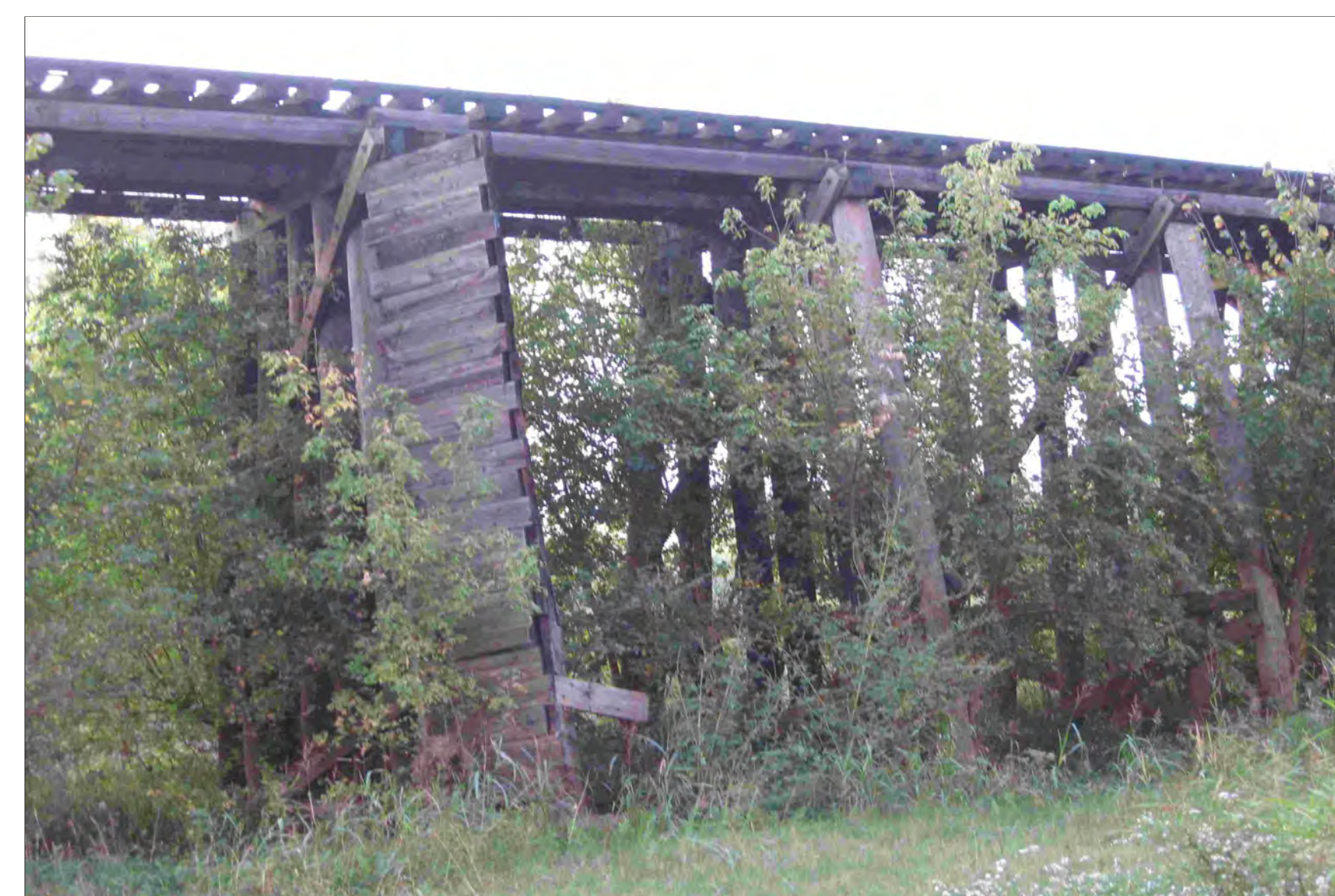
ATSF Wood Trestle Segment
